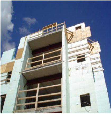
Window and Door openings are also prepared during build using permanent or temporary buck materials which will support concrete during placement. Once at projected wall height, vertical reinforcing steel is inserted into wall cavity as specified. Concrete placement is recommended using boom pump and internal vibration to assure even placement and monolithic pour condition.
